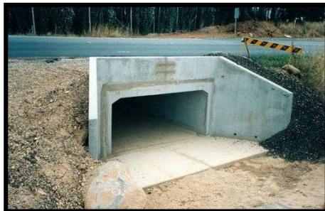
Typical pre-formed box culvert
