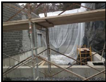
New wall for clarifier building
