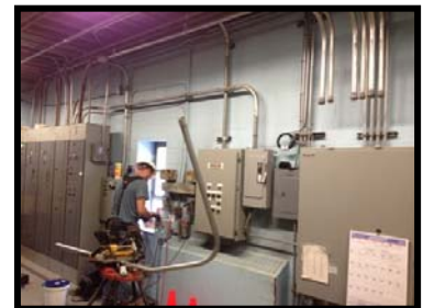
Conduit installation at plant
