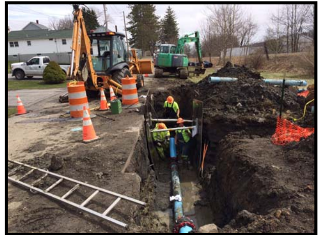
Borough crews complete work lowering a water main
