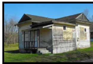
Mine 42 First Aid Station
