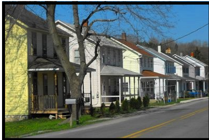
Mine 42 Company Houses
