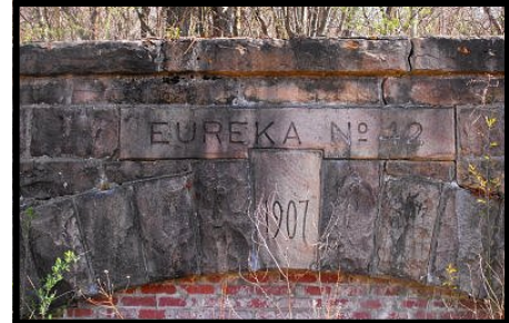
Sealed Mine 42 Portal
