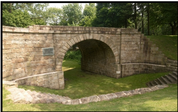
Allegheny Portage RR Skew Arch Bridge
