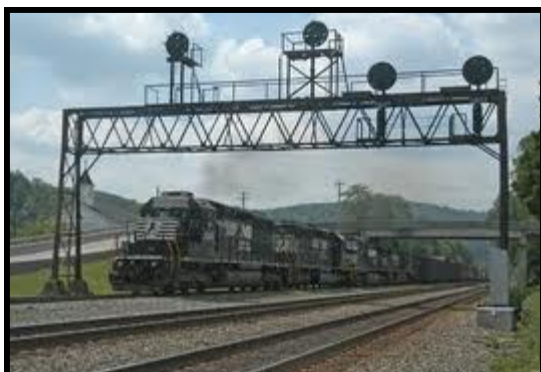
Summerhill Bridge and Signal Tower
