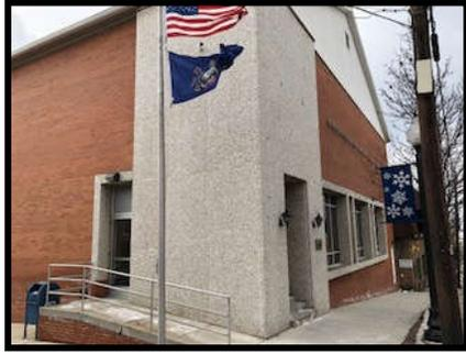
Second, the white aggregate panels will be chemical washed. The rusted fasteners will be replaced, and holes filled. Area will be sealed. (\$6,630)
