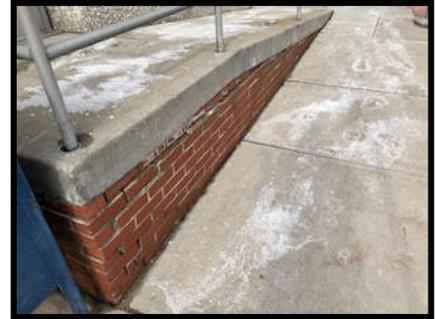
Third, the lower portion of the front and side walls, approximately four feet high, has many spalling bricks. Those will be replaced as necessary. The mortar joints will be repointed. All will be sealed. (\$7,850)
