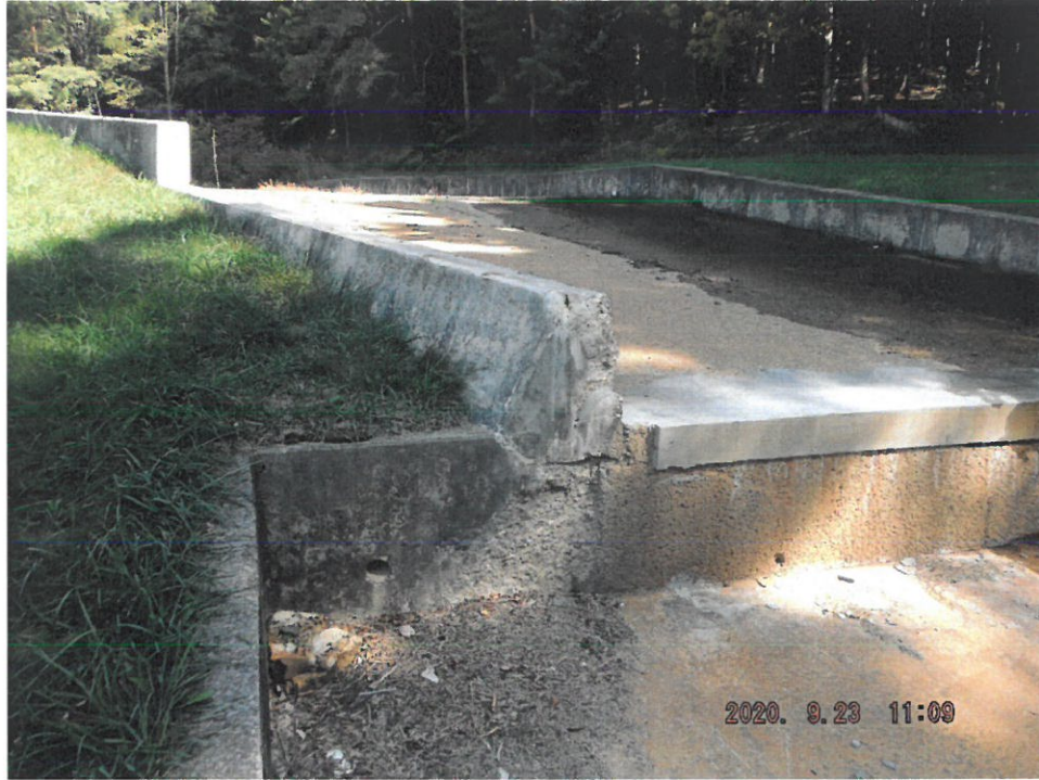
Photo 13: Recently Removed Upper Section of the Western Spillway Wall (EMA operational staff removed portion of wall in 2019)
