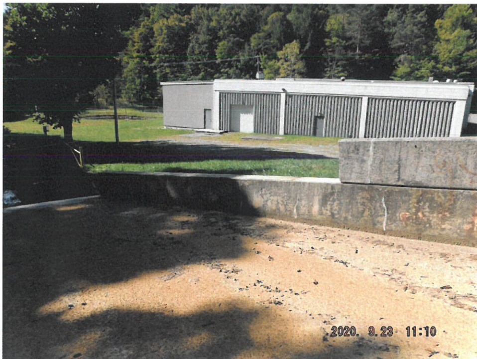
Photo 18: Recently Removed Upper Section of the Western Spillway Wall (EMA operational staff removed portion of wall in 2019)
