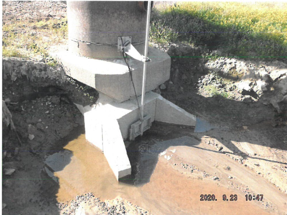
Photo 17: Newly installed primary closure drain valve. (20" Stainless Steel Sluice Gate)
