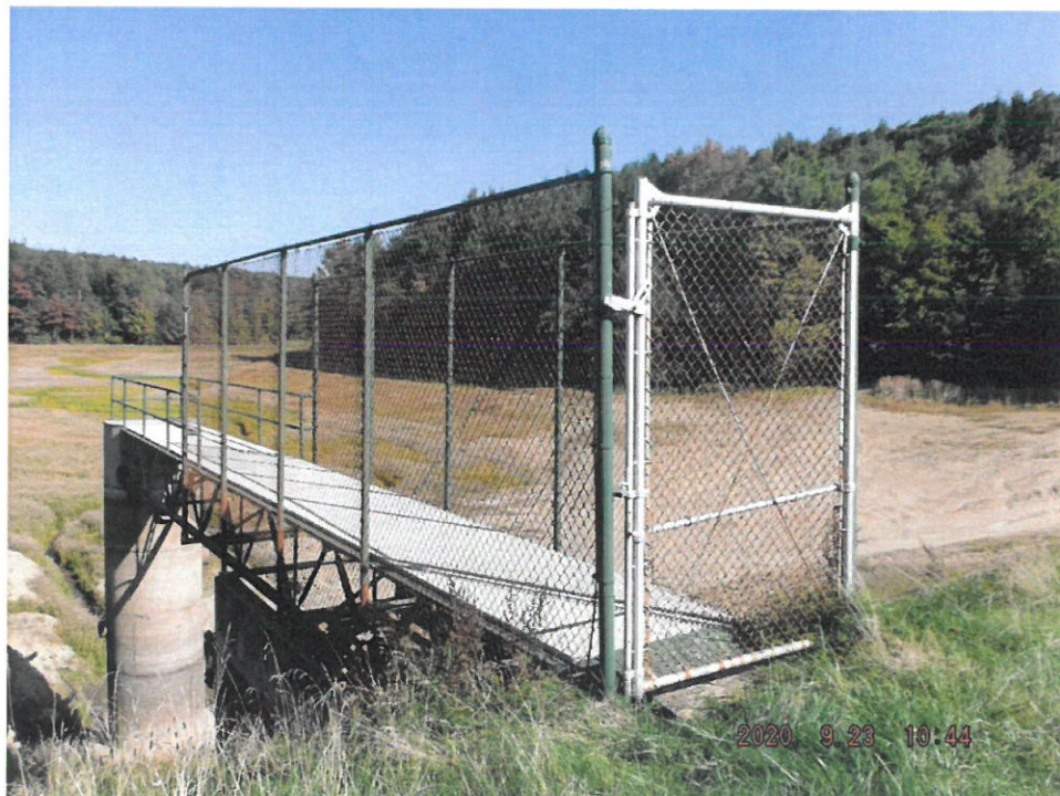
Photo 4: Intake Structure, Bridge and Gated Access
