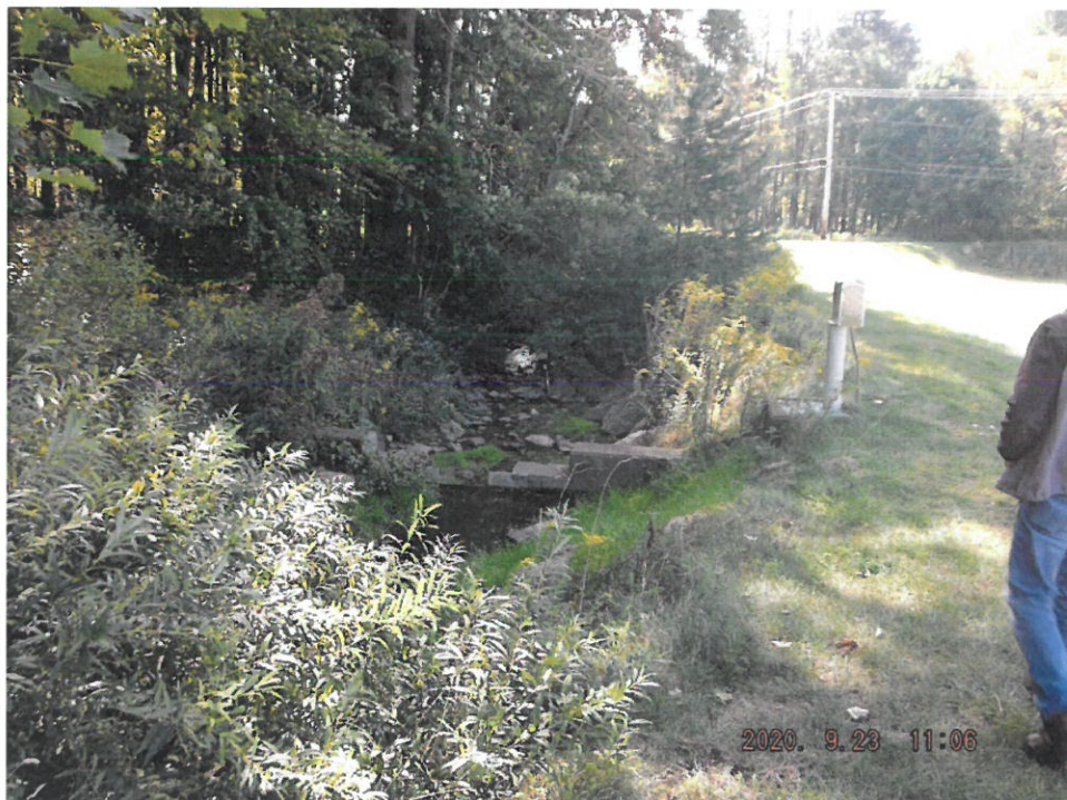
Photo 12: View of Weir on Discharge Channel Used for Measuring Conservation Release
