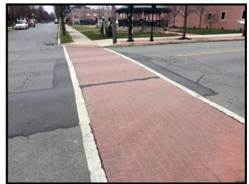
Those same tires cause a depressed path in the adjacent blacktop. Since the concrete does not wear in the same way, the blacktop becomes lower than the concrete, causing tires to hit the edge of the crosswalk hard. In 2015 borough crews made repairs to the blacktop surfaces to smooth the transition to the crosswalks. The concrete crosswalks have also suffered significant cracking, and borough crews keep those cracks sealed.
