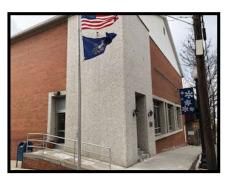
Second, the white aggregate panels will be chemical washed. The rusted fasteners will be replaced, and holes filled. Area will be sealed. (\$6,630)
