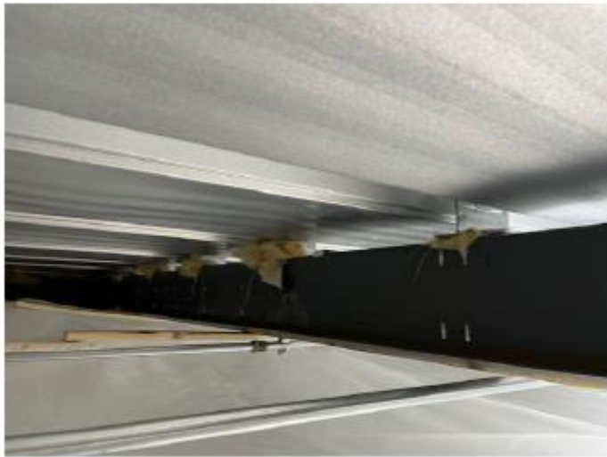
← Area where insulation was removed
