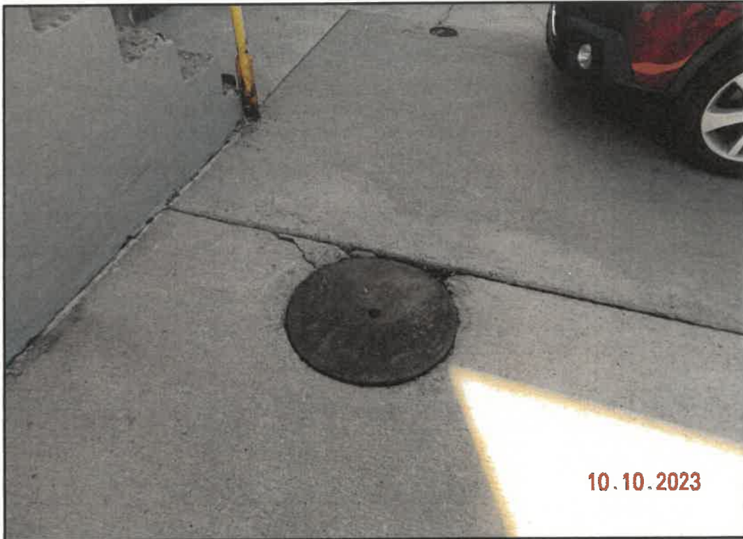
Photo 15: View of Reservoir Drain Manhole
