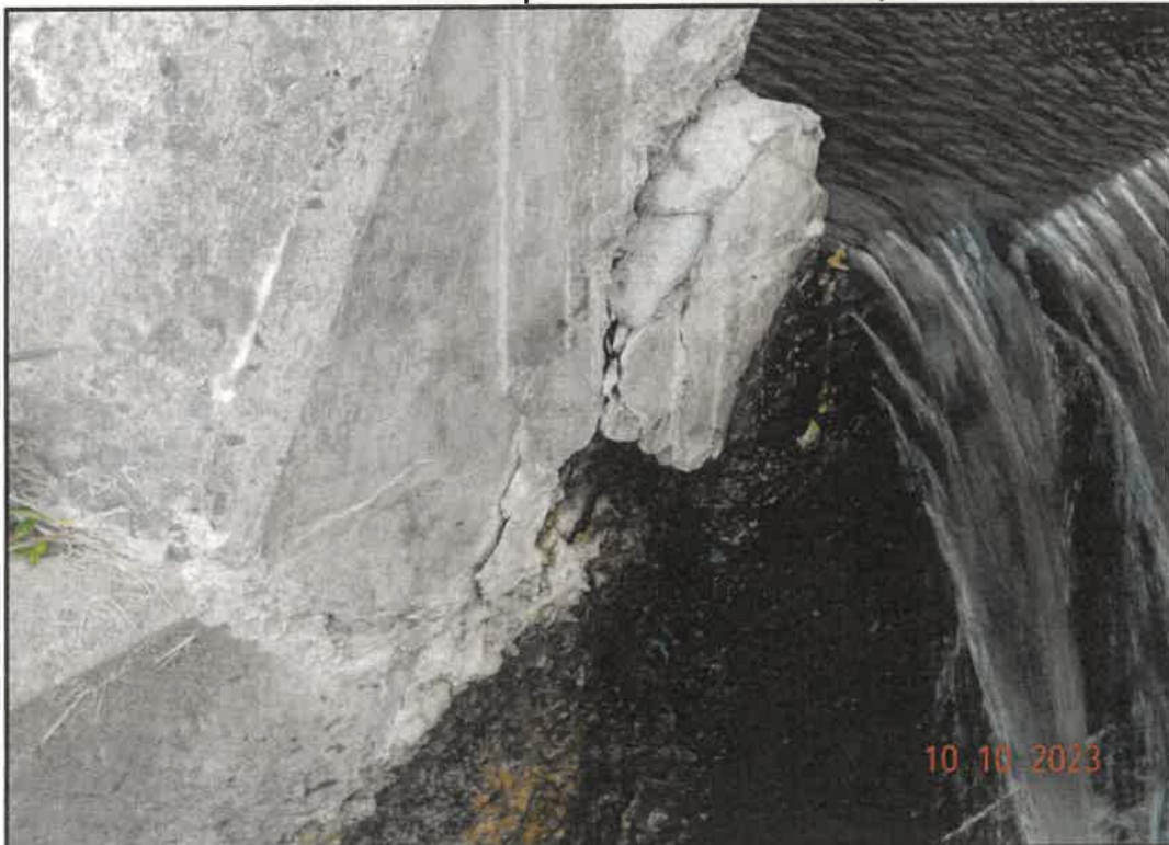
Photo 14: Portion of downstream spillway channel patched/repared by EMA operational staff in 2019
