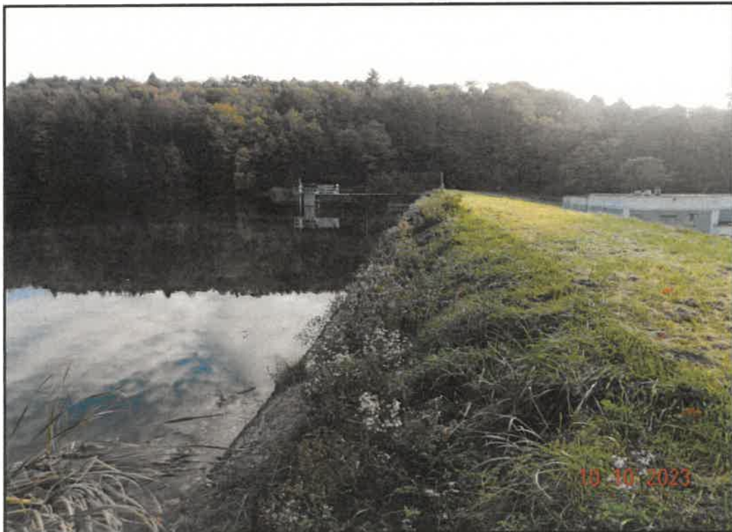
Photo 2: Upstream Embankment looking Northeast
