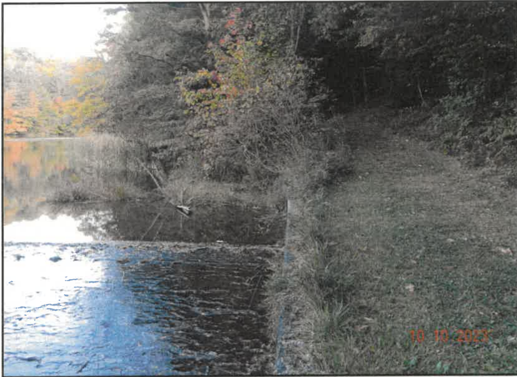
Photo 9: Woody Vegetation at East Abutment
