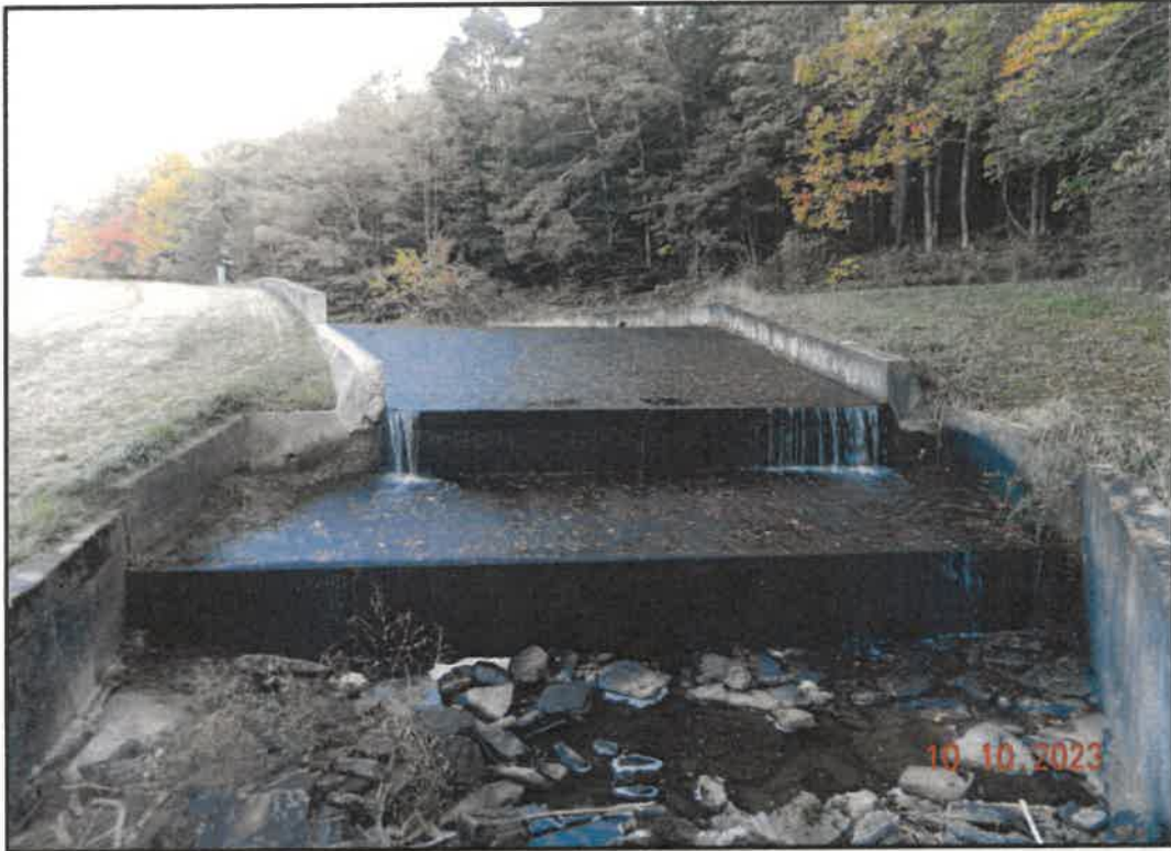
Photo 11: Downstream Section of Spillway
