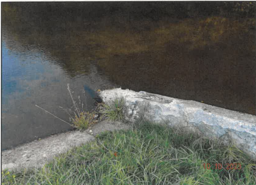
Photo 8: Spillway Control Section looking Northeast
