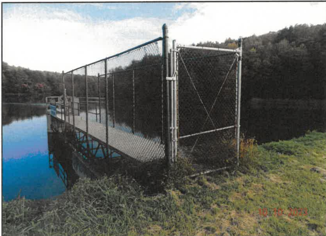
Photo 4: Intake Structure, Bridge and Gated Access
