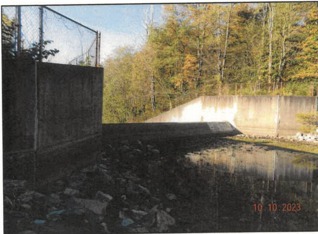
Photo 10: View of Spillway Weir and Walls
