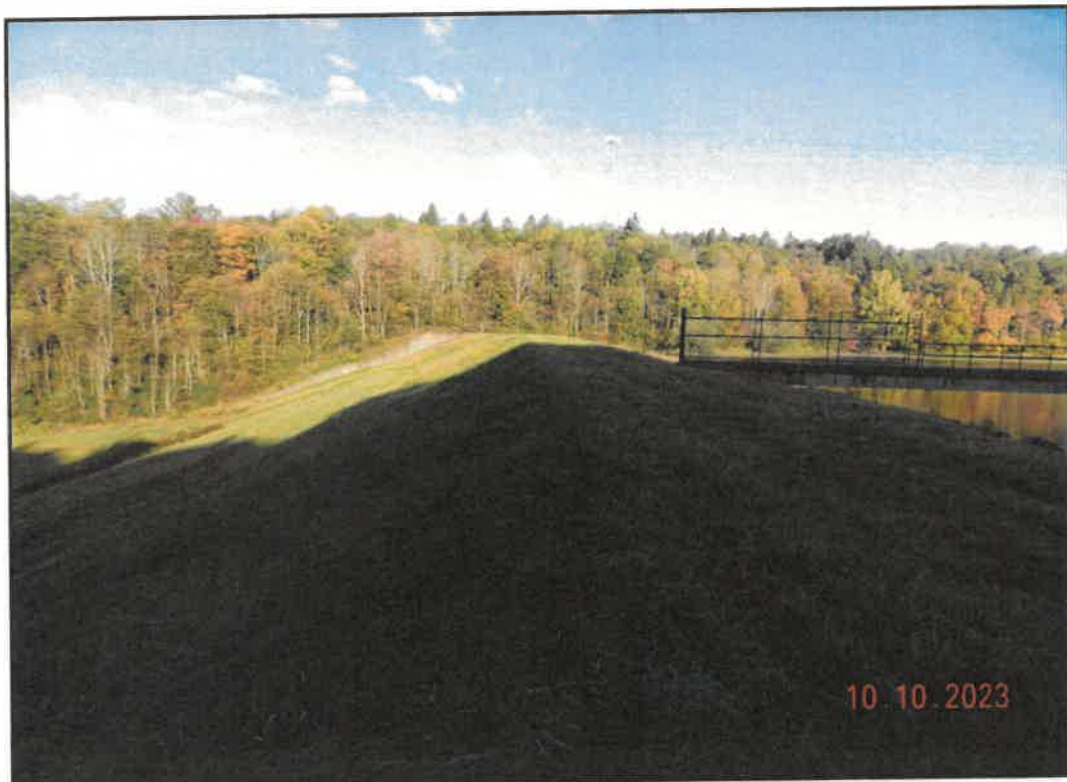
Photo 2: Downstream Embankment Looking Northwest
