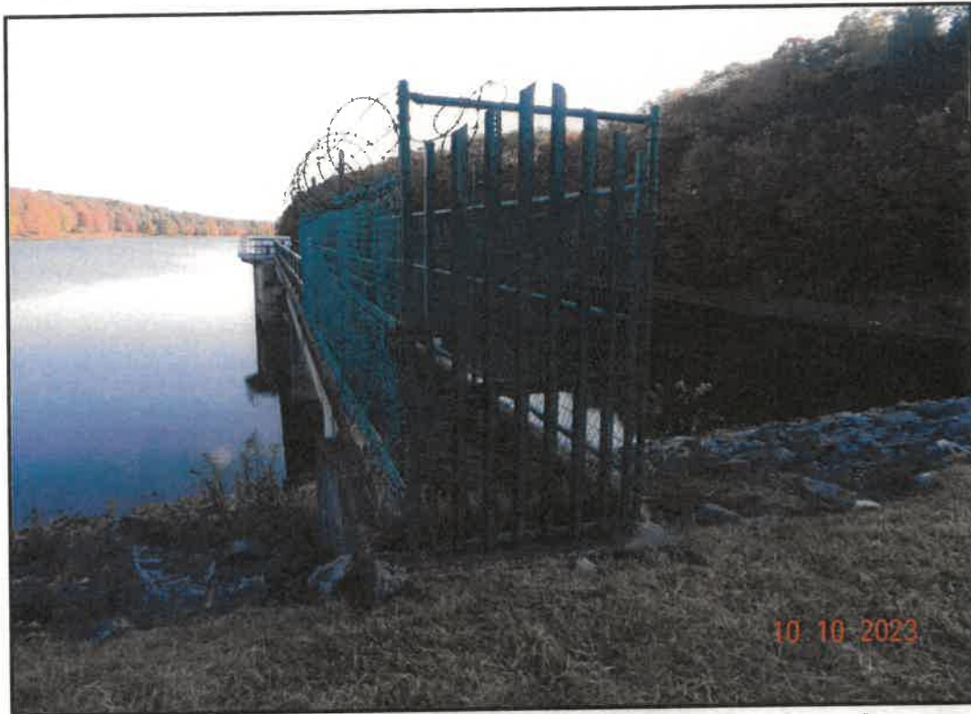
Photo 5: View of Locked Gate Access to the Bridge and Intake Structure
