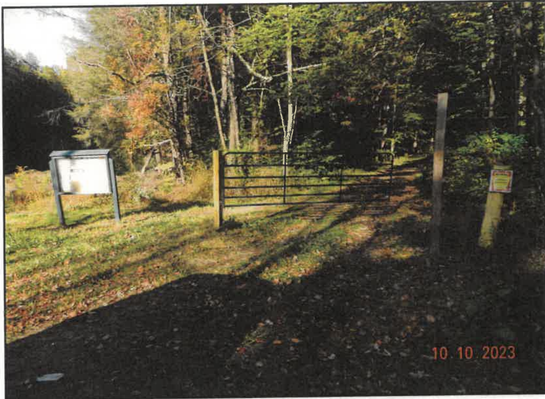
Photo 1: View of Gated Access to Dam
