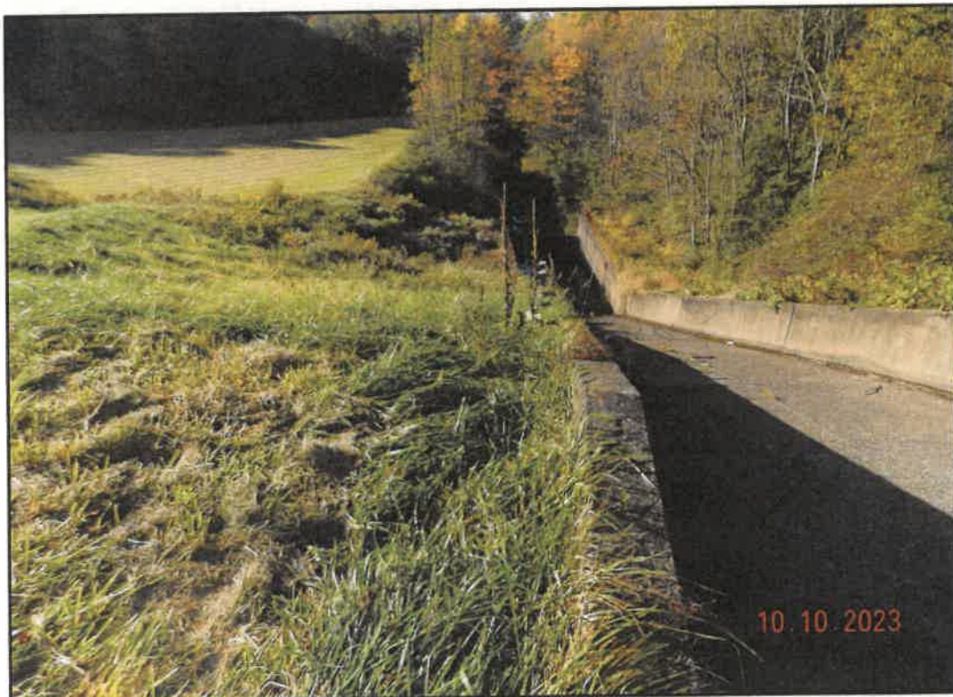
Photo 14: View of Eastern Spillway Wall
