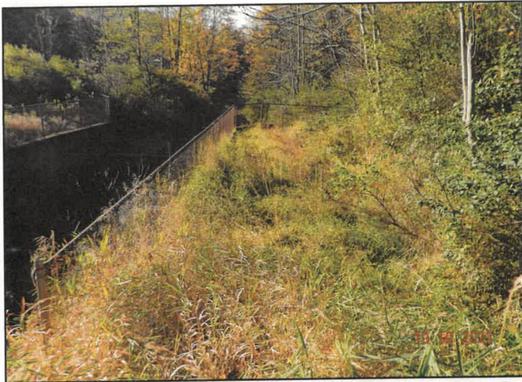
Photo 31: View of Wet Area behind Western Abutment Wall at Stilling Basin
