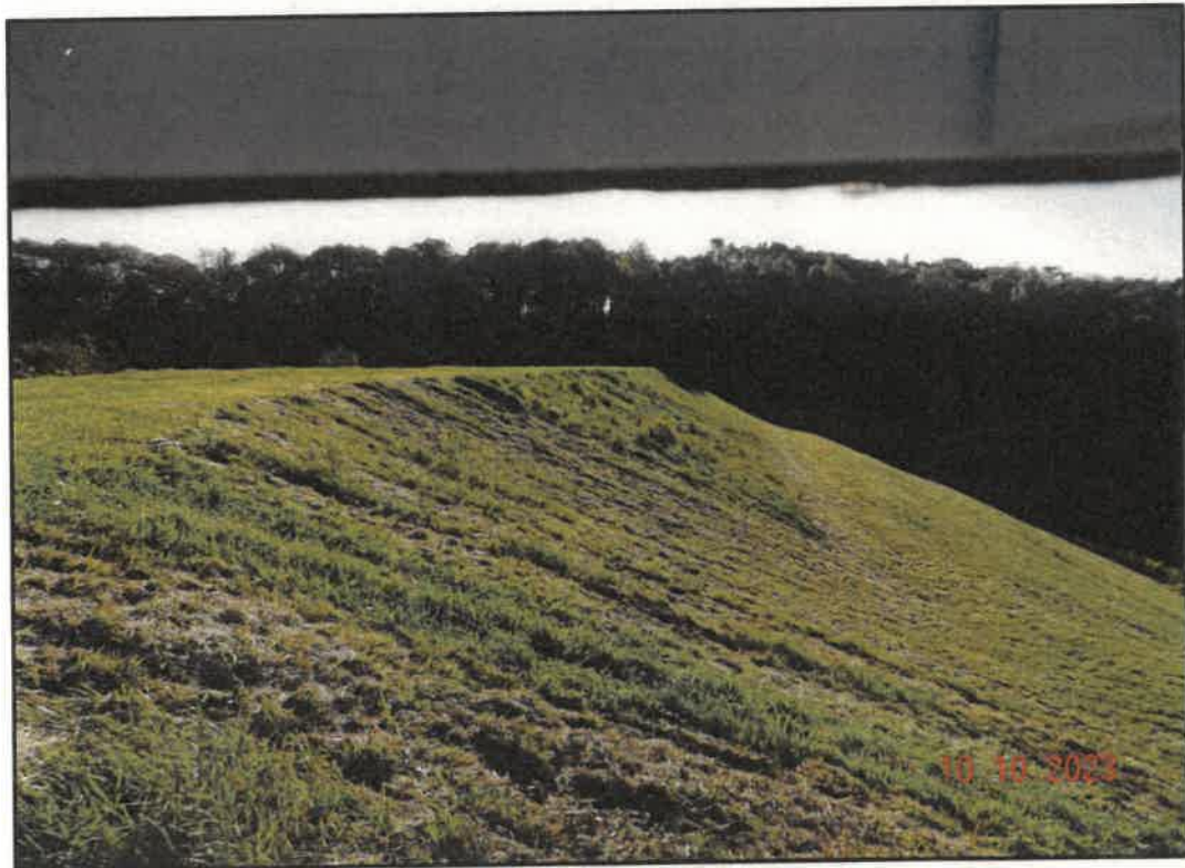
Photo 12: Downstream Embankment looking Southeast
