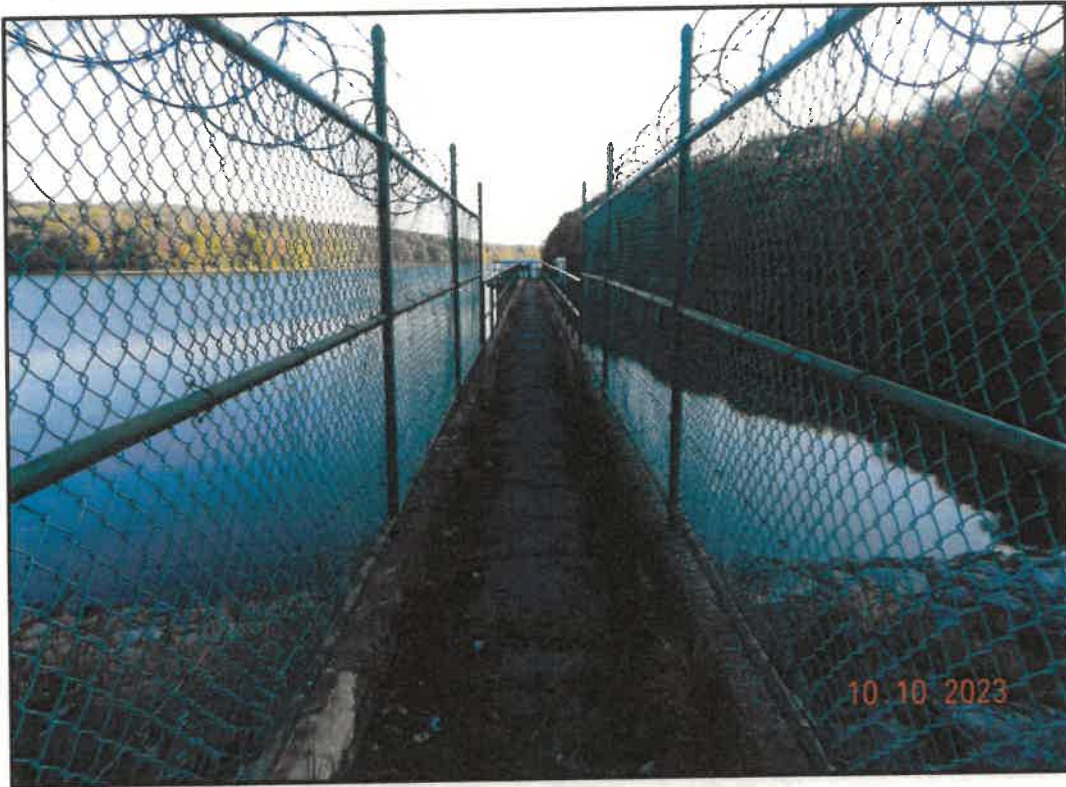
Photo 7: View of Bridge Walkway
