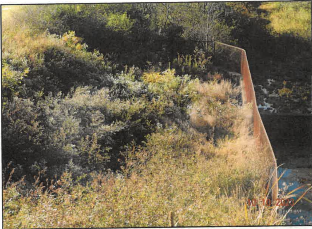
Photo 27: View of Wet Area behind Eastern Abutment Wall at Stilling Basin
