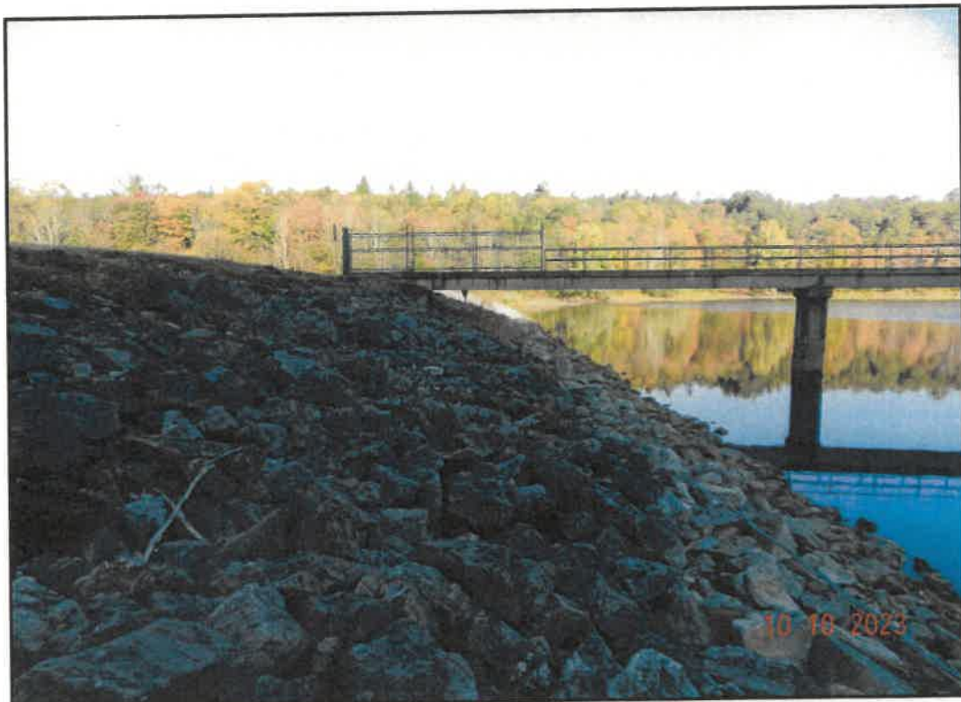
Photo 4: Upstream Embankment looking Northwest
