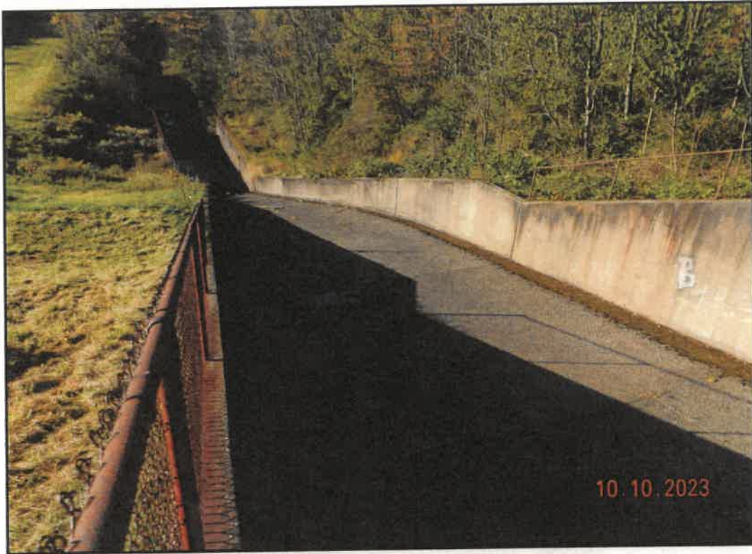
Photo 11: Spillway Channel looking South
