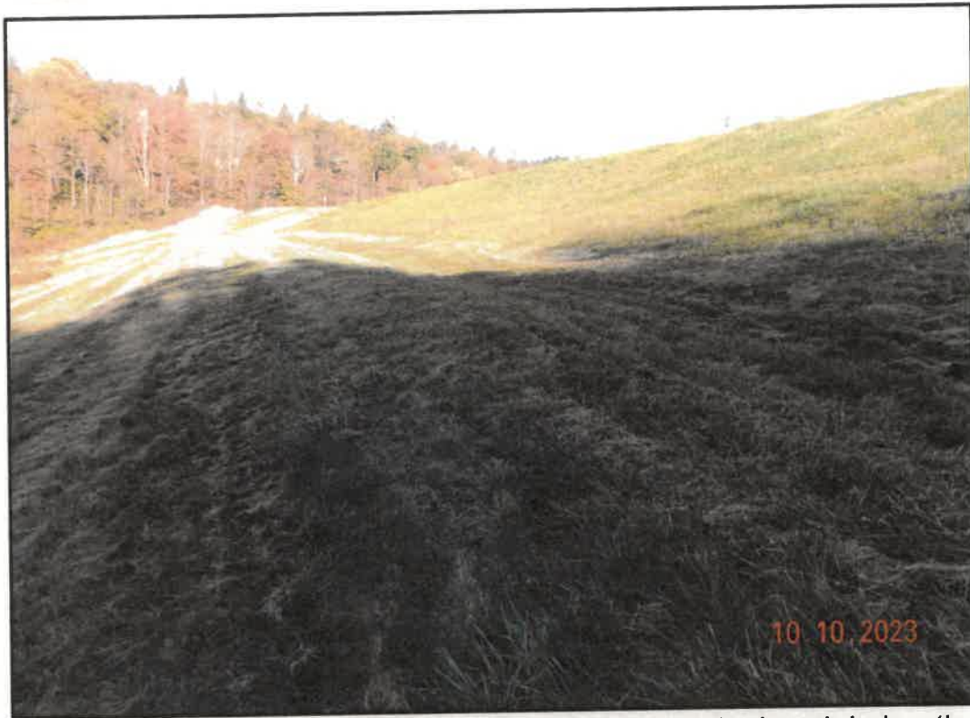
Photo 23: View of Typically Wet Area (dry this year) on the 1st bench below the Dam's Crest. This view is typical for the majority of the crest.
